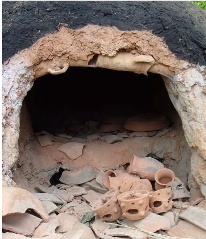
Fig. 5. Reusing waste jars in building the roof of the kiln, yogurt jars sticking out the ceiling are recycled ones and an environmental aspect, Climbing kiln, Khomeir Mahale, Amlash, Ali Ashraf Babaie (Ziaee, 2016)
